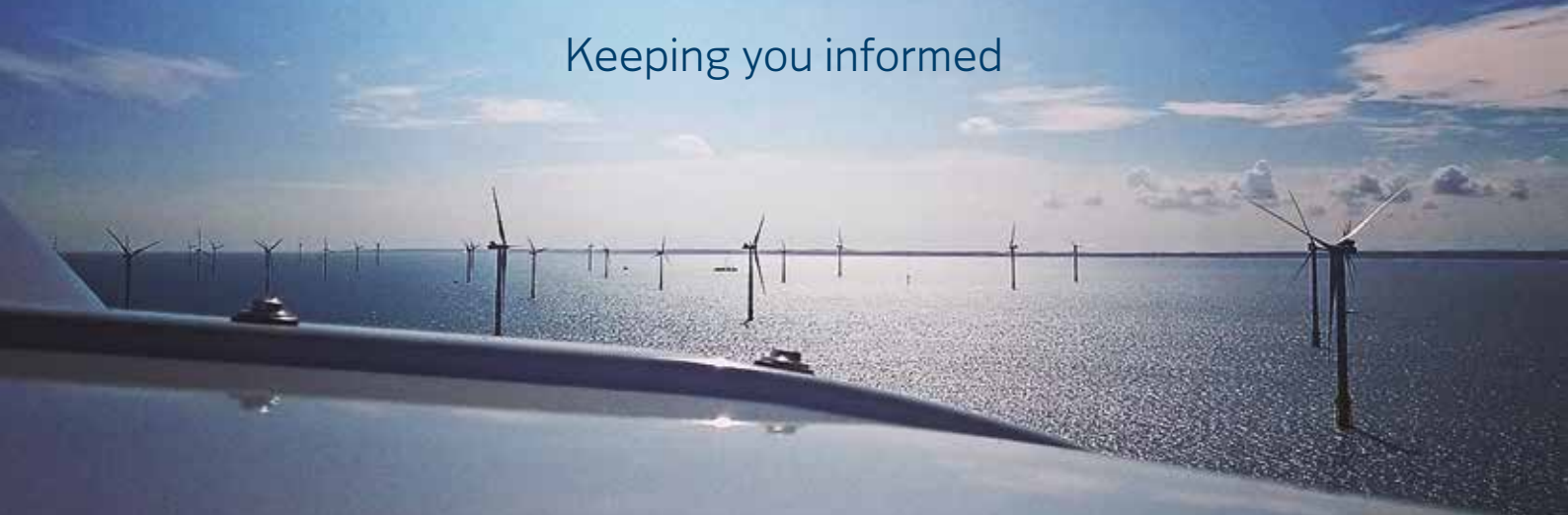
Thanet Offshore Wind Farm
