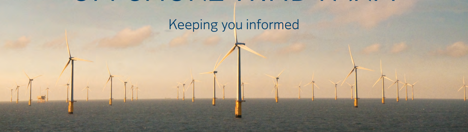
Thanet Offshore Wind Farm
