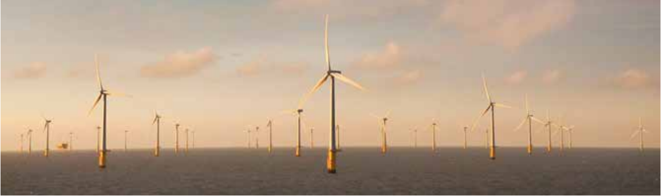
Thanet Offshore Wind Farm
